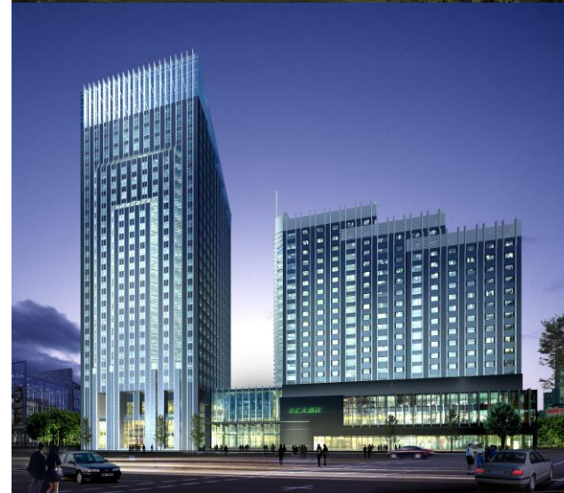
山西正韵 Shanxi Zhengyun City Commercial building project
