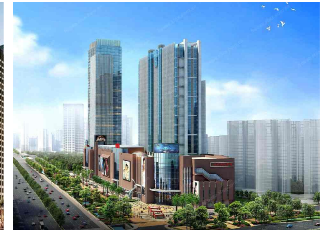
Foshan Shibo Plaza Project
