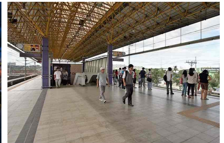
Philippines LRT-2 Rail Project
