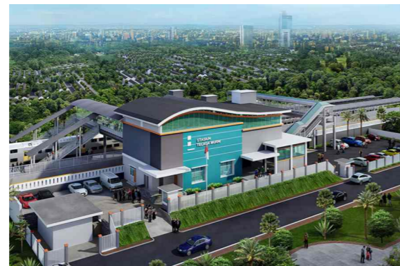
Indonesia Metland Telaga Murni Station Project
