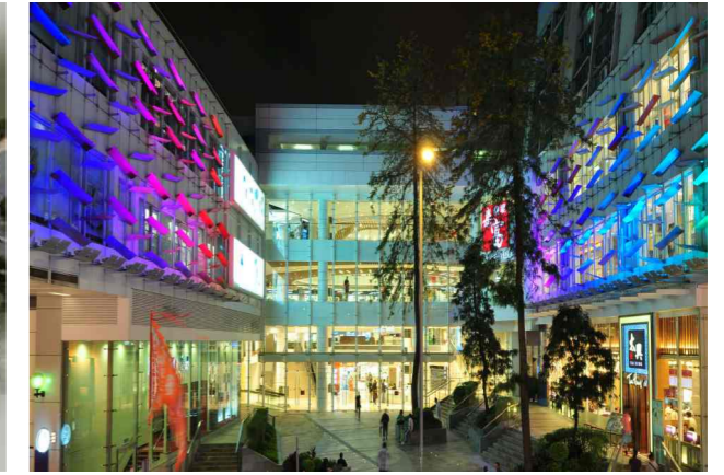
Hong Kong Lok Fu Shopping Center Project
