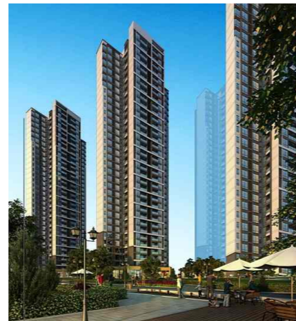
Guizhou Wuxingxingang Estate Project
