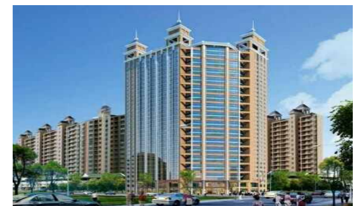
蚌埠市固镇棚户区改造安置房 Bengbu Gu Town Resettlement House
